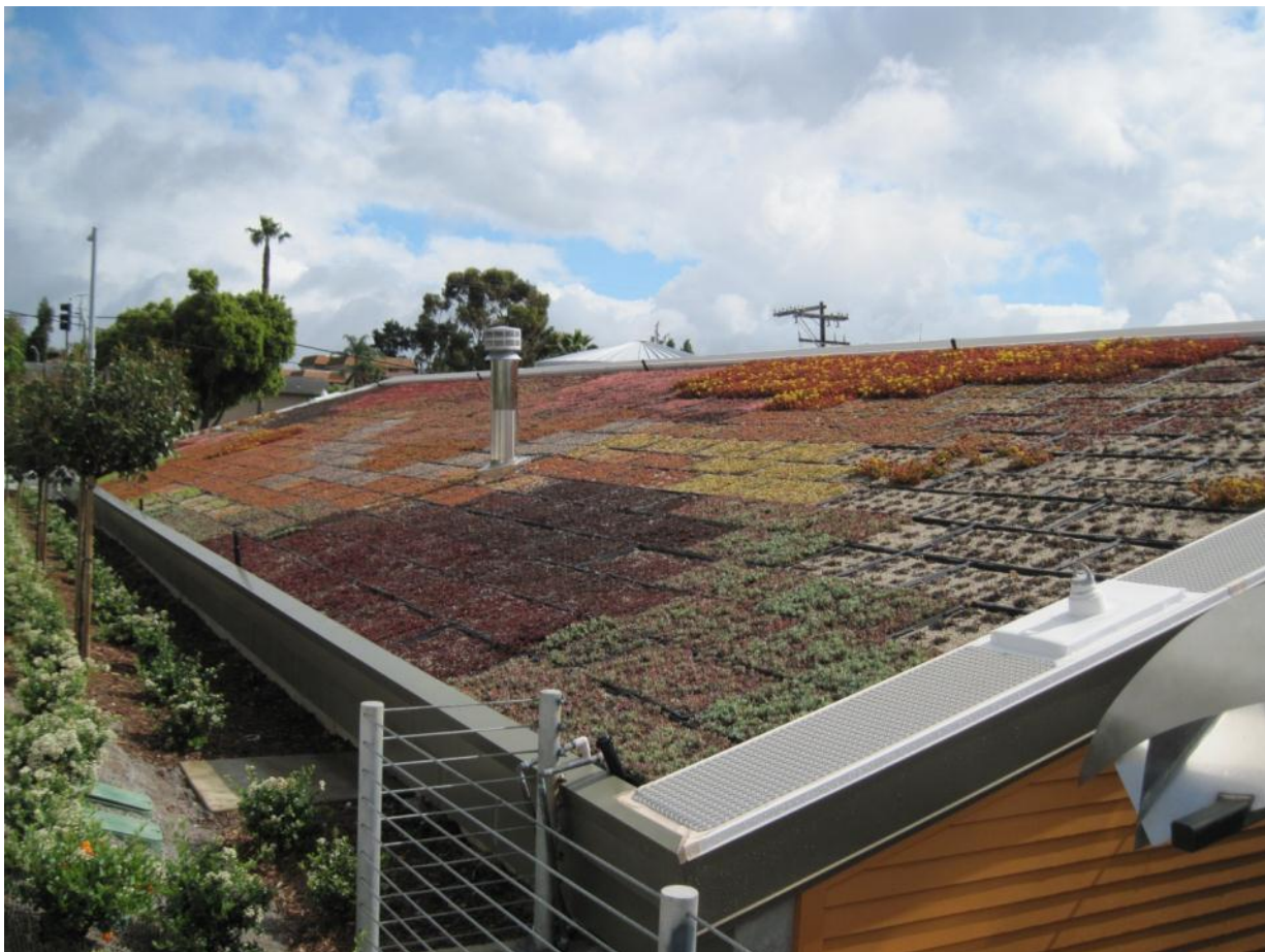
Figure A.6-2. Extensive vegetated roof.
